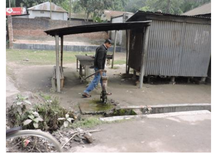
Fig 3.18: Tube well facility
