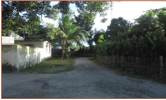
Fig 3.2: Narrow and Poor Upazila Road
