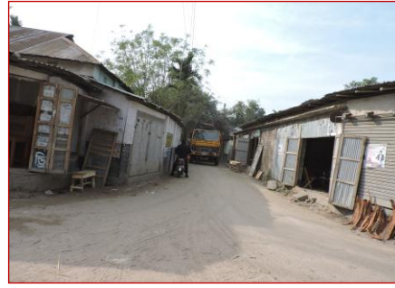
Fig 3.3: Narrow and Poor Upazila Road
